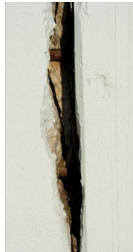
Figure 2.47 MINIMALLY ACCEPTABLE floodwall. Exposed surface rebar resulting from poor construction practices. The public sponsor has painted over the rebar in an attempt to keep it from rusting. (MN)
