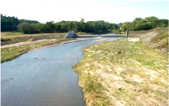
Figure 2.70 UNACCEPTABLE channel shoaling below a control structure. The original channel bottom extended all the way to the riprapped banks. There is an estimated 2-3 feet of sediment in the channel, mostly from upstream field erosion and highway construction. (MN)
