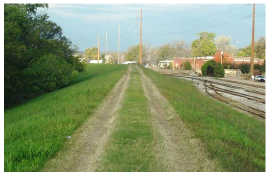
Figure 2.39 UNACCEPTABLE rutting in levee. (OK)
