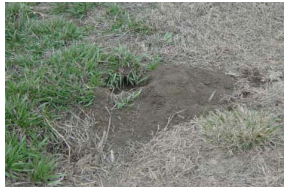
Figure 2.20 Animal burrow in a levee. (IA)
