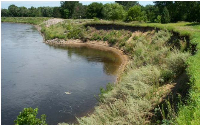
Figure 2.24 Channel erosion located at the upstream end of a flood control levee protected by riprap. Erosion caused by riprap protection and eddy currents. (MN)
