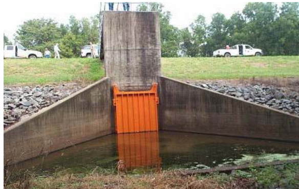
Figure 2.63 ACCEPTABLE culvert gate. (LA)
