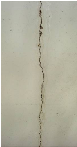
Figure 2.43 MINIMALLY ACCEPTABLE 1/8 th inch crack extends through concrete floodwall and needs to be sealed to prevent further damage. (MN)
