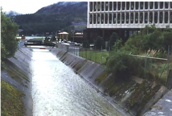
Figure 2.74 ACCEPTABLE concrete lined channel. (AK)
