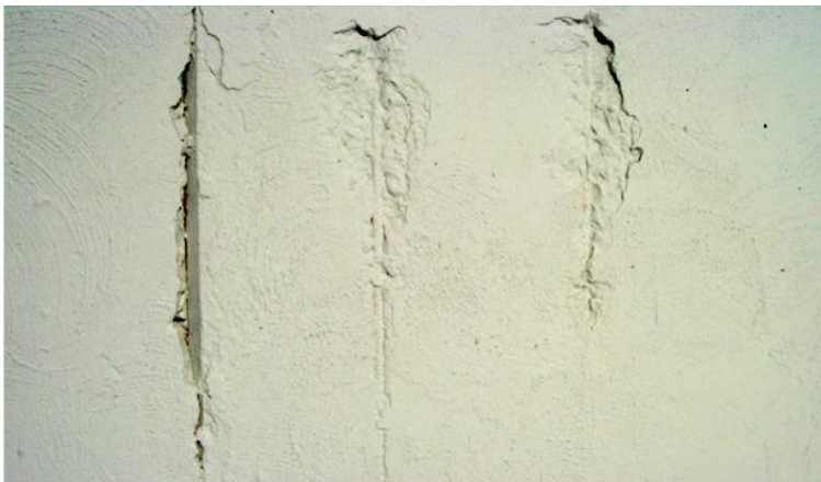
Figure 2.47 MINIMALLY ACCEPTABLE floodwall. Exposed surface rebar resulting from poor construction practices. The public sponsor has painted over the rebar in an attempt to keep it from rusting. (MN)
