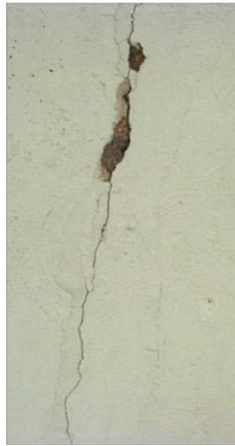
Figure 2.44 MINIMALLY ACCEPTABLE Vertical floodwall crack with spalling. The rating for this particular crack is Minimally Acceptable because the crack is still tight but there is some spalling occurring as well. (MN)
