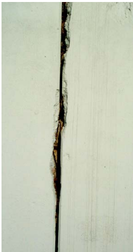
Figure 2.45 UNACCEPTABLE exposed rebar. Monolith joint separation with exterior spalling along the joint and interior spalling in the area of the rebar. (MN)
