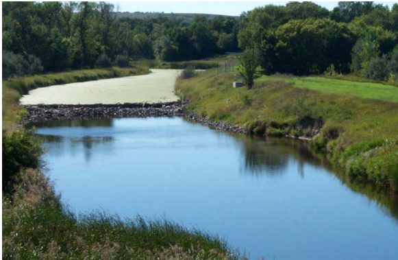
Figure 2.15 UNACCEPTABLE. Slope failure and erosion caused by inadequate channel bottom and side slope protection. This was a direct result of bottom scouring that undercut the levee slope and erosion caused by turbulent flow at the end of the bank protection. (ND)
