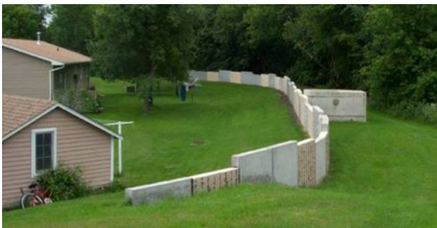
Figure 2.48 MINIMALLY ACCEPTABLE floodwall. Monolith joint separation caused by settlement, no landward or riverward tilting. The opening is about 3 inches wide at the top but the rubber joint sealer is still intact and undamaged. This joint has since been repaired by bolting another joint sealer on the both sides of the wall and filling the void with an expandable joint sealer. (ND)
