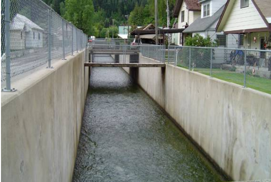
Figure 2.72 ACCEPTABLE concrete lined flood control channel. (ID)
