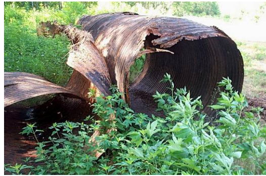
Figure 2.62 Pieces of the same pipe, once removed from the levee. Note that while much of the pipe may have appeared to be in good condition from the inside, the outside was extremely corroded. The public sponsor attempted to patch the pipe the first year, but when it failed again, the entire CMP was replaced.
